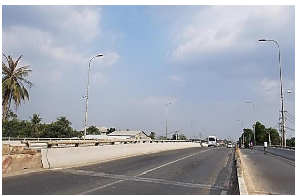
LED lighting system supplied and installed by Vietnam-Schreder & SAPULICO companies on Highway 22 Tp. Ho Chi Minh - Tay Ninh. Total power of HPS lamps: 295.075 kW, total power of LED lamps: 207.131 kW; The amount of electricity saved per year: 379.918 kWh.
