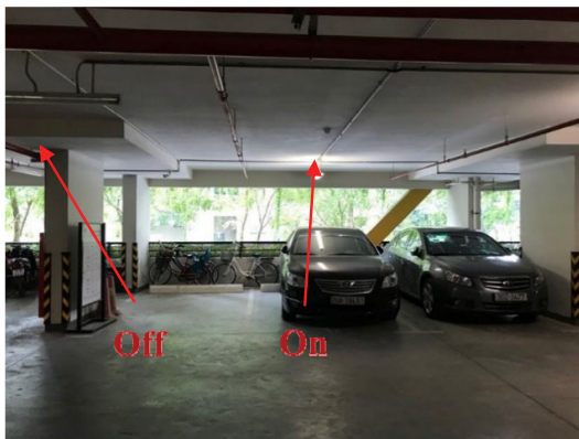
Figure 2.14. The lighting system near the wall is staggered on and off
