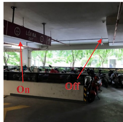
Figure 2.14. The lighting system near the wall is staggered on and off
